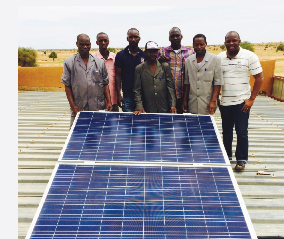
Newly installed solar panels
